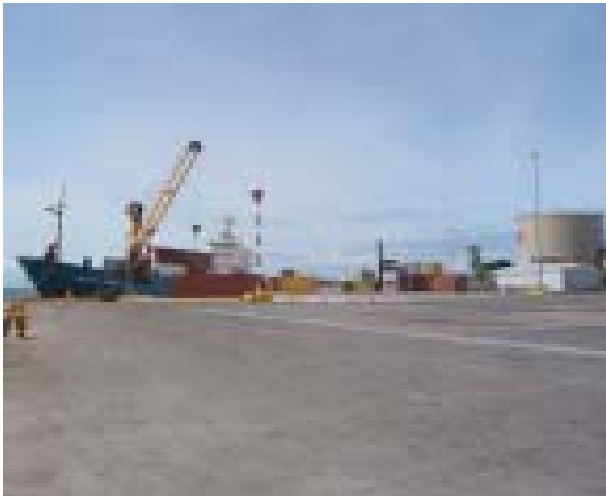
New Extension to the Apia Wharf
