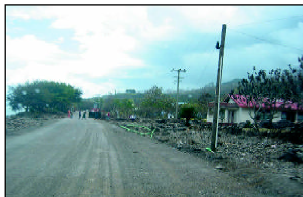
Road repair at Luatuanuu after Cyclone Heta
