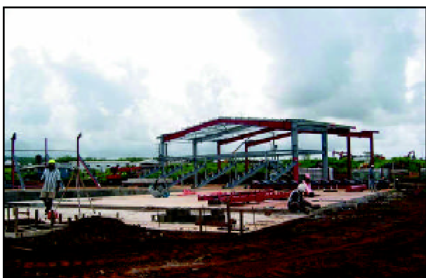
Construction of new sports complex at Tuanaimato
