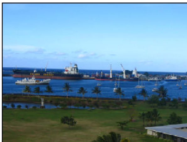
Apia Wharf extension allows more berthing space for large vessels
