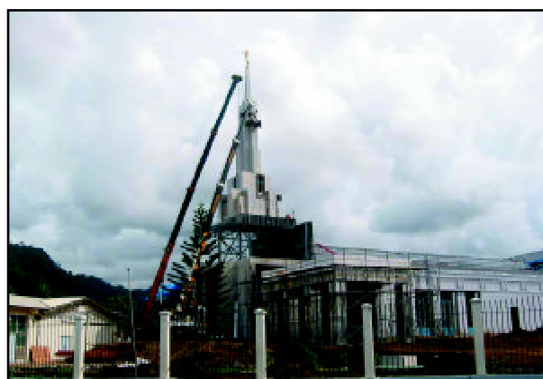
New LDS Temple at Pesega under construction
