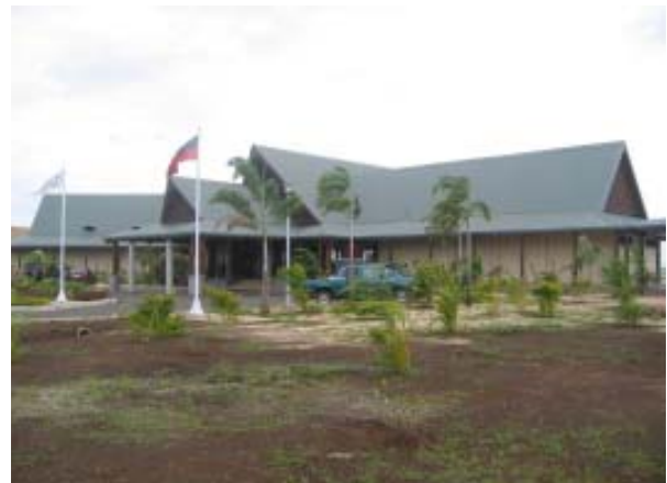
Complete Phase I of the Aggie Grey's Lagoon Beach Resort and Spa, Mulifanua
