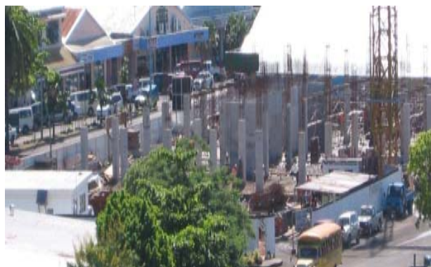
Development Bank Headquarters under construction.
