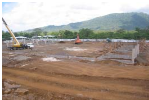
Foundation for the new Gym No. 2 at the Tuanaimato Sports Complex.
