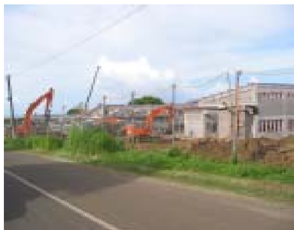
New buildings for the National University of Samoa, Le Papaigalagala.
