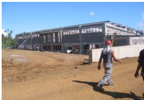
New buildings for the National University of Samoa, Le Papaigalagala.
