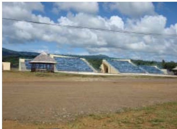
Construction of new Beach Volleyball facilities at the Tuanaimato Sports Complex.
