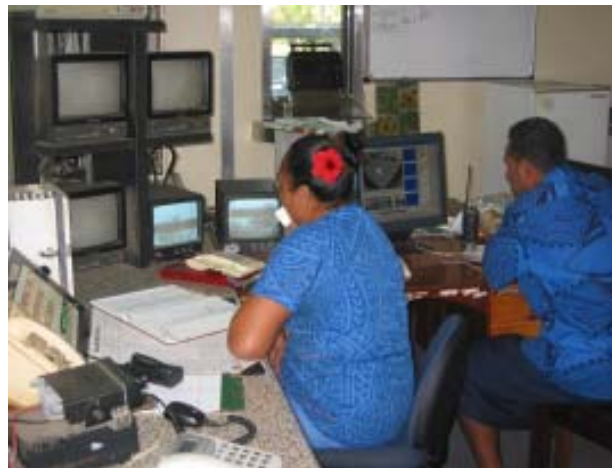
Upgraded security system in the Guard Room.
