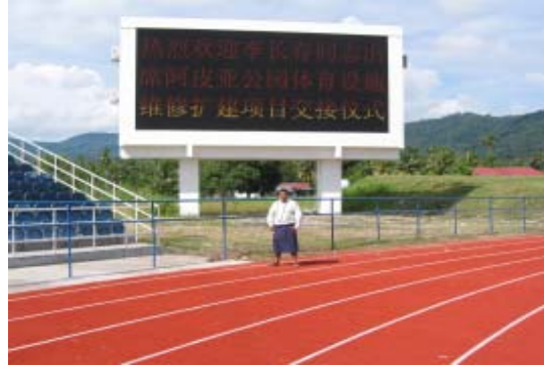
Apia Park Stadium near completion
