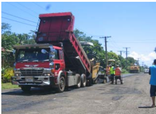
Road repair works after heavy flooding in February 2006.
