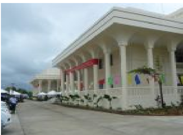
The completion of a major construction project, the Courts of Samoa and Ministry of Justice Building, which was officially opened on 25 January 2010.
